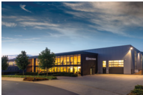
Manufacturing centre in Leopoldshöhe
